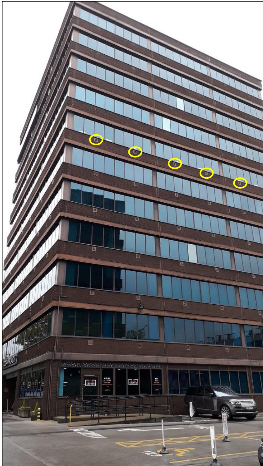
Figure 1: South elevation to 1 City Approach showing five (5) of the twenty four (24) passive ventilation grilles on the 6 th Floor.
