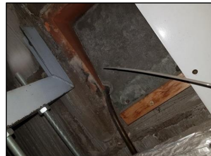
Figure 9: Restricted/obstructed passive fresh-air vent/
