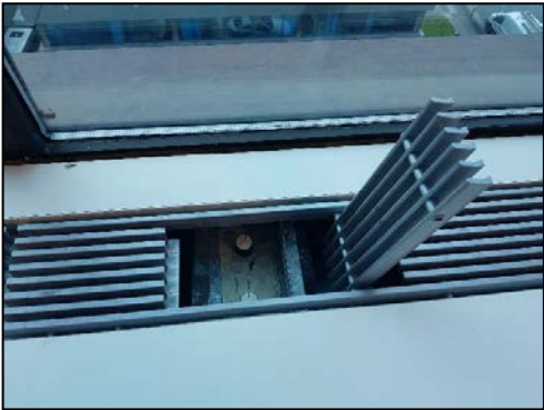
Figure 4: Fan Coil Unit control potentiometers.
