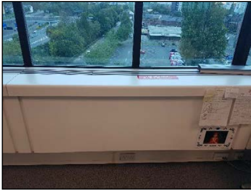
Figure 2: Fan Coil Unit with external cover installed.
